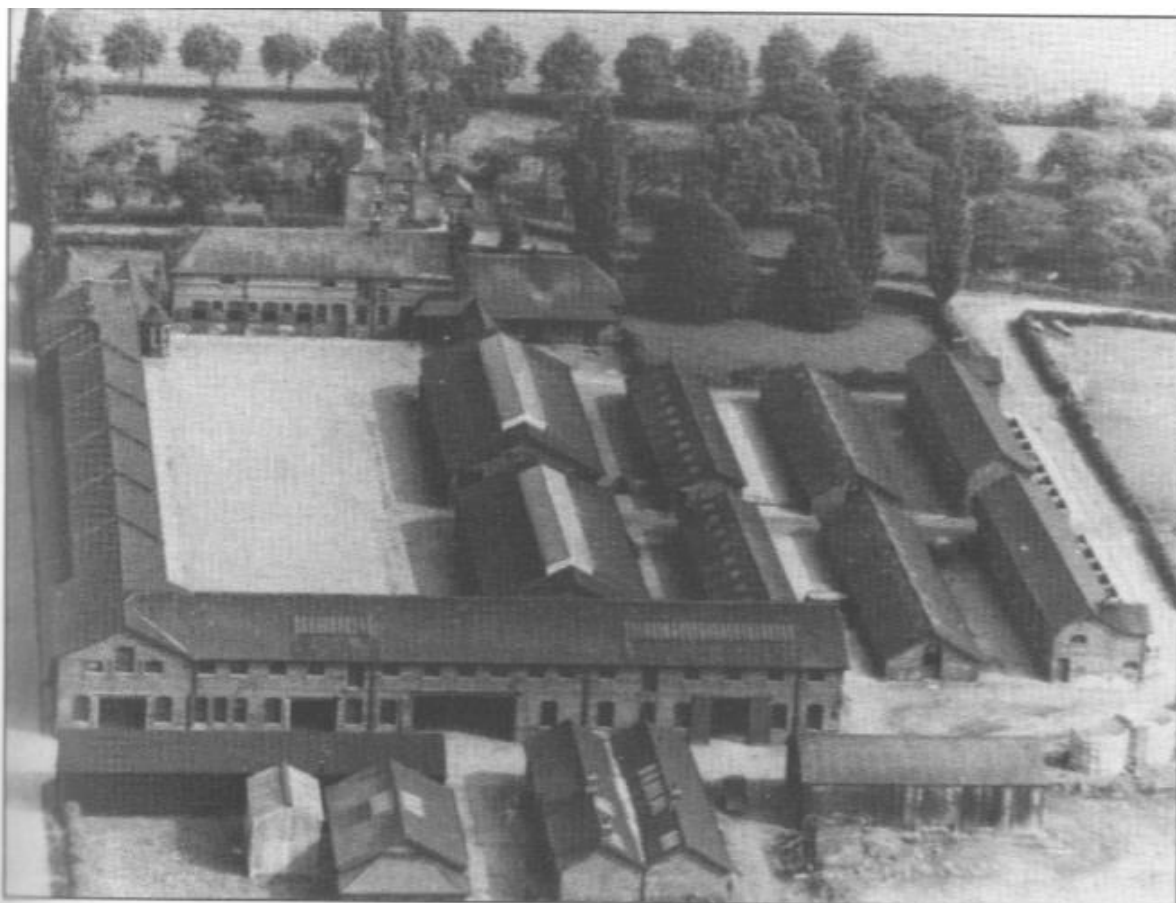
An aerial view of Bulcote Farm buildings
